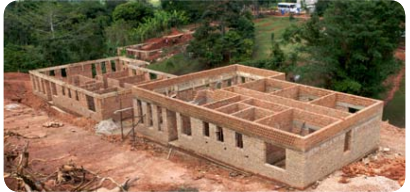
Construction of houses 8 & 9
